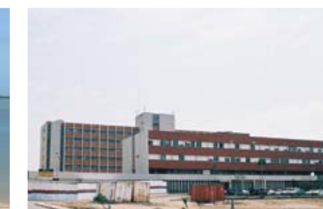
Hospital do Lubango | Lubango
